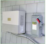
Sharp's 3.5kW inverter is designed with a neutral-toned NEMA 3R housing that integrates into the look of almost any style home.
